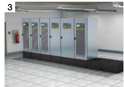
3 30 minutes later: 800 kW, online double conversion mode
