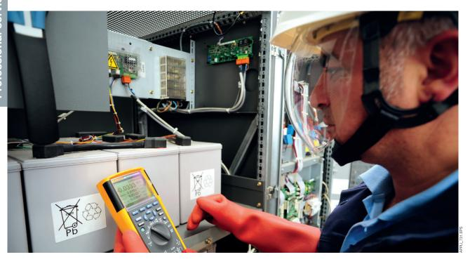
The Power Quality Audit (PQA), is a service offered by Socomec that checks the load level and the quality of the low voltage electrical installation.
